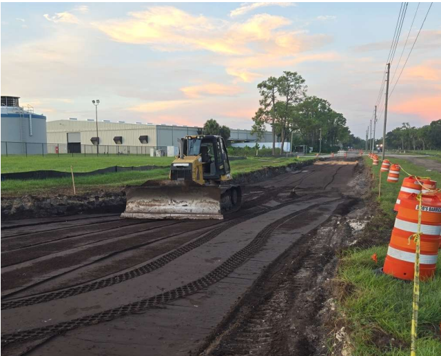
Webster Turn construction
